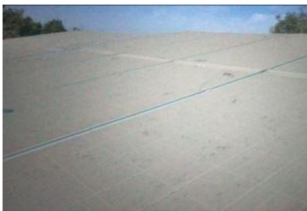
Solar Panels affected by dust accumulation (Before)
